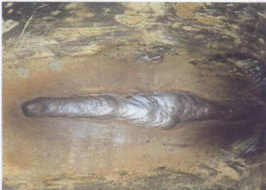
Point after welding.
