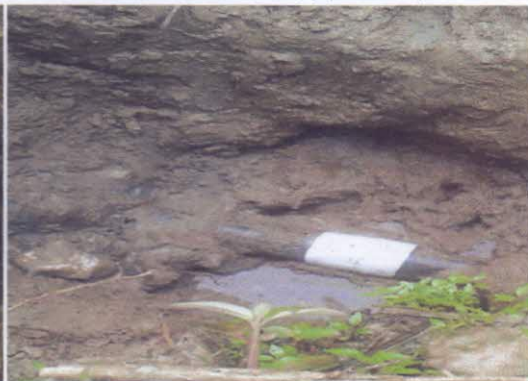
Point after rapping ready for backfilling.
